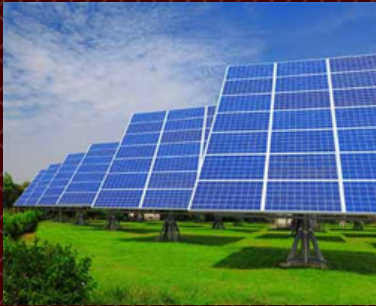
SOLAR PANEL & SPARES
